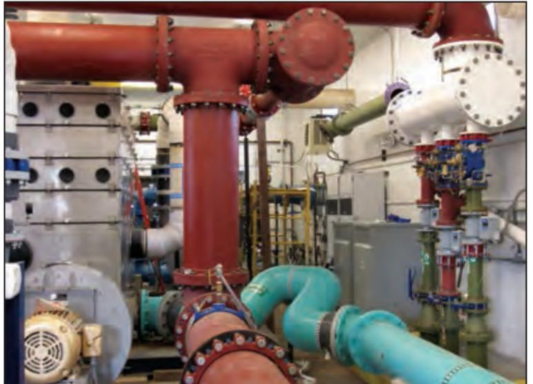
The effluent pipework through which the water flows after PFC treatment.
