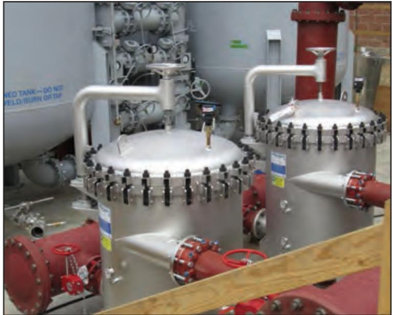
Above and below, different views of the prefilters that remove sediment from raw water brought into the water treatment system.
