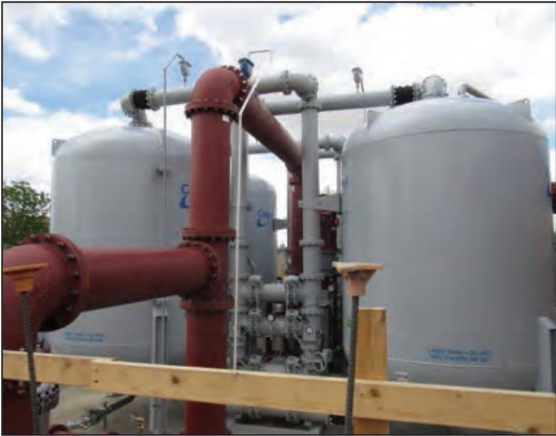
Influent raw water is piped into these large PFC treatment vessels.
